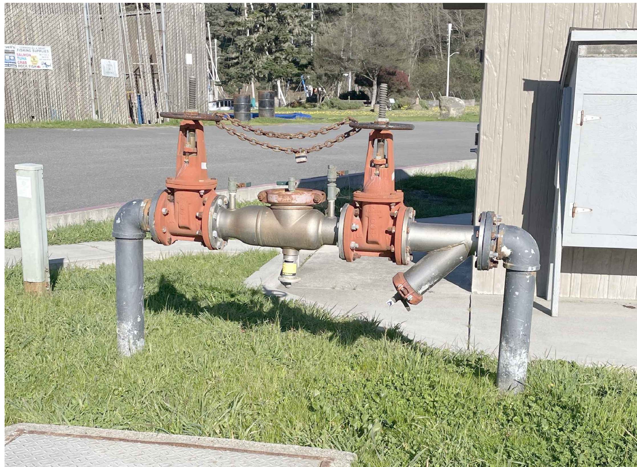
DETAIL 4 NTS (BACKFLOW PREVENTER)
